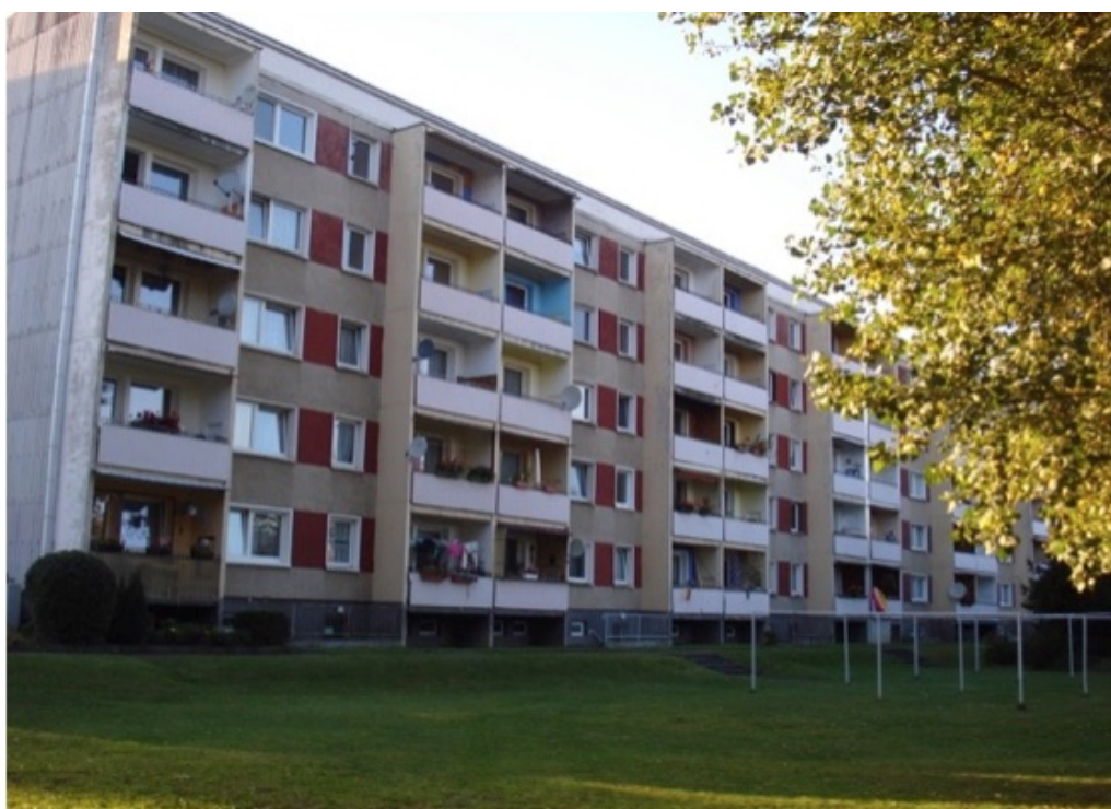
FIG. 2. Prefabricated buildings dominate Genthin Süd.
